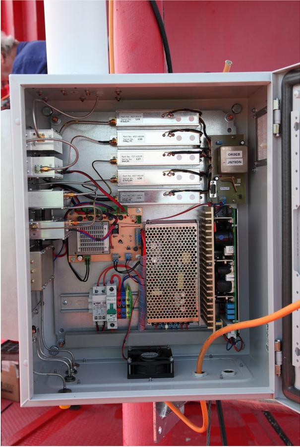
The image shows the interior of a white metal electrical cabinet. On the left side, there are three stacked power supply units (PSUs) with labels. A black cooling fan is mounted at the bottom center. Various colored cables (red, blue, green, black) are connected to the units. On the right side, there is a green control unit labeled 'OK0EB - JAVTRON'. The cabinet is open, and the background shows a red wall and a person's shoulder. |
